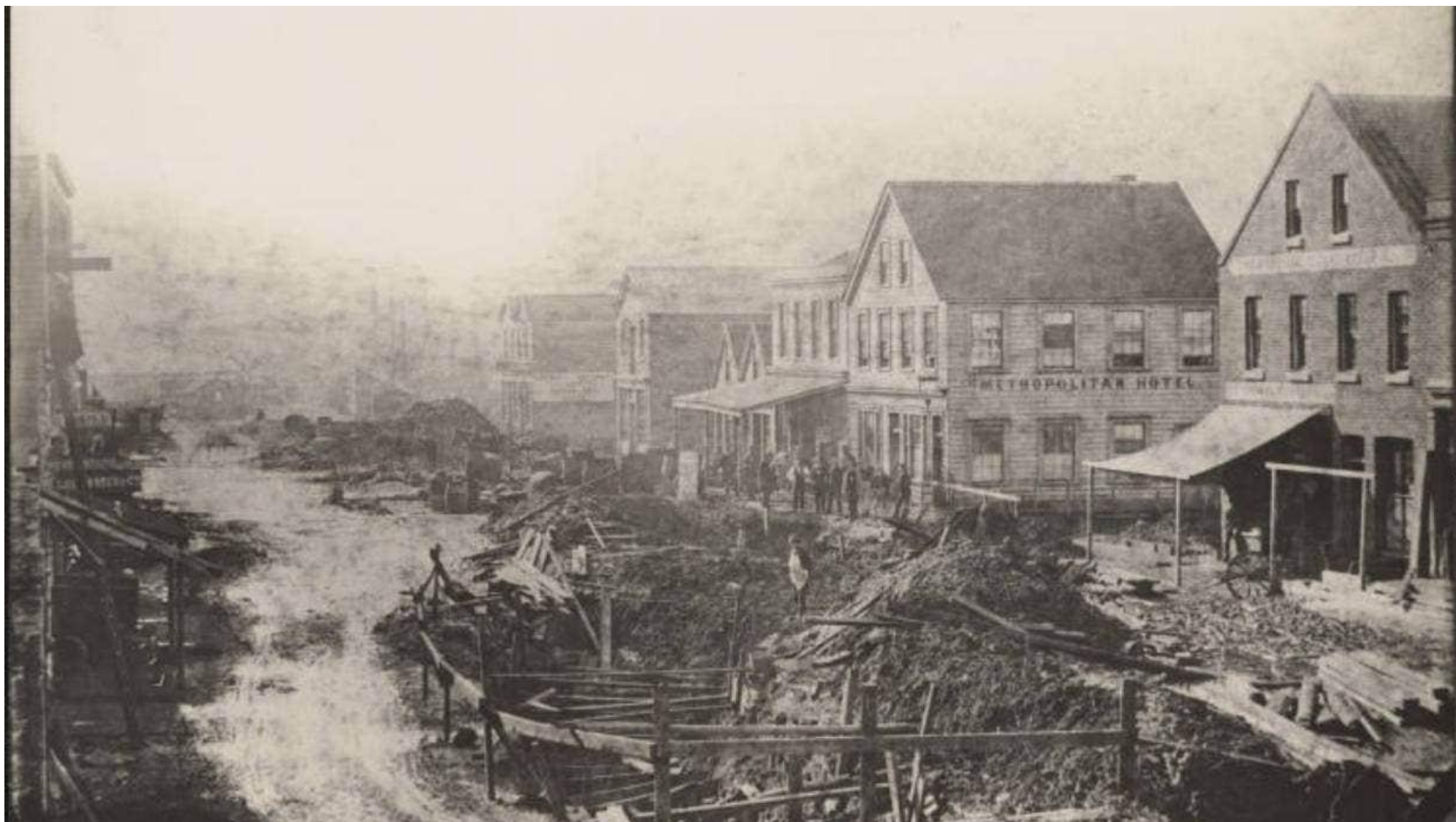
Queen St sewer built around Waihorotiu in 1860. Auckland Libraries Heritage Collections
